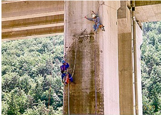
Figure 4-12 Special Inspection of a pier
