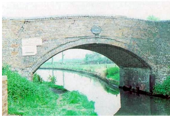
Figure 4-10 Cracking of a spandrel wall of a masonry arch bridge
