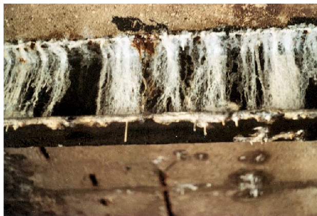
Figure 4-4 Efflorescence on steel girders due to leakage through concrete deck
