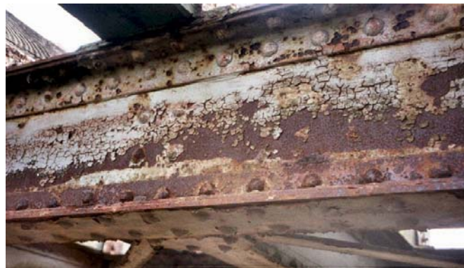
Figure 4-9 Corroded steel superstructure
