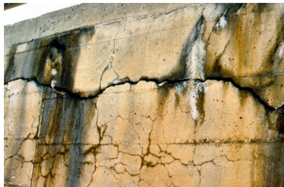
Figure 4-8 Cracking of a concrete wing wall due to ASR
