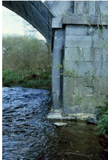
Figure 4-3 Bulging of a masonry abutment due to excessive earth pressure
