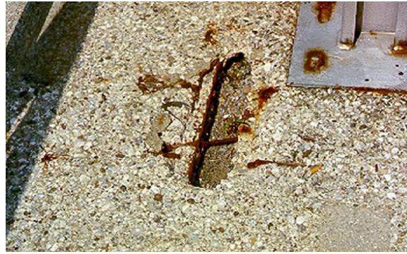
Figure 4-5 Freeze-thaw damage of a footway aggravated by the action of de-icing salts
