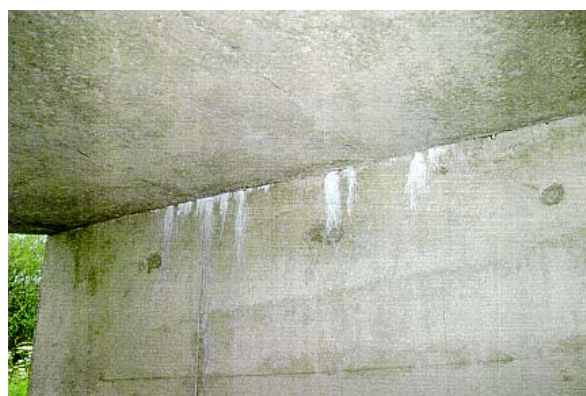
Figure 4-2 Deterioration of the construction joint between the roof and side wall of a concrete box structure due to differential movement
