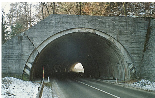
Figure 4-6 Cracking of a tunnel portal and vault due to foundation instability
