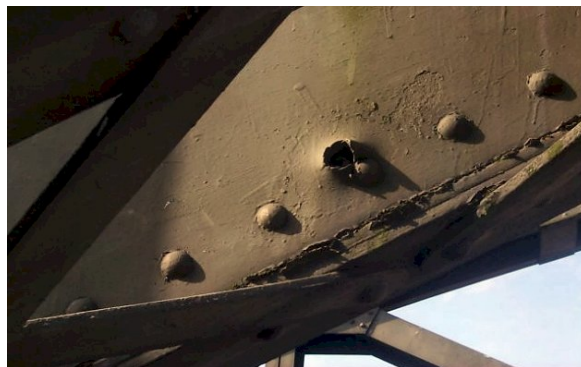
Figure 4-11 A bullet hole in a steel structure
