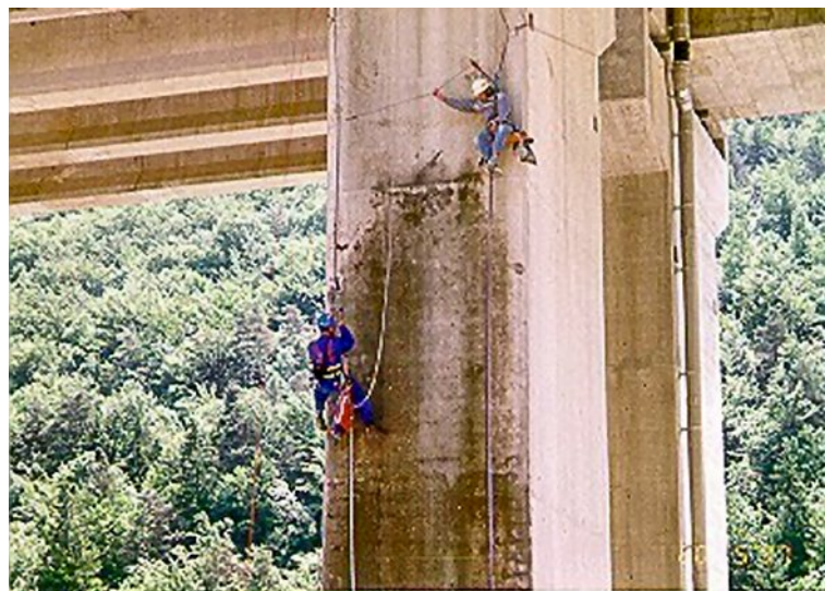
Figure 4-1 Special Inspection of a pier
