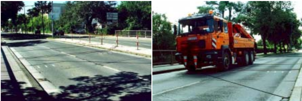
Figure D.7: Pneumatic axle detectors on the road surface
