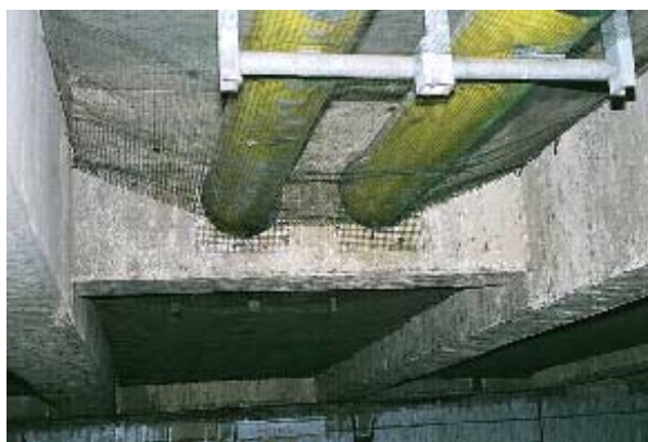
Figure D.3: Views of the bridge from below, 3 rd field
