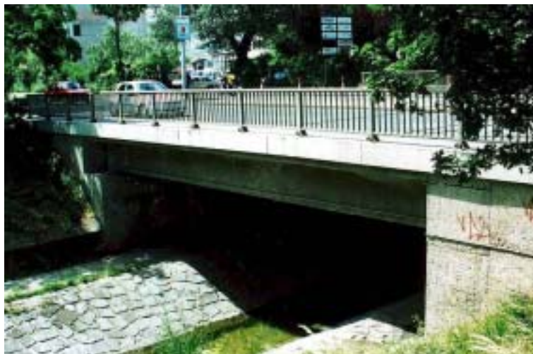
Figure D.1: Investigated bridge in Vienna
